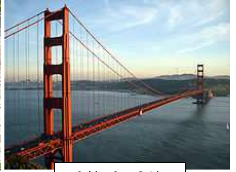
Golden Gate Bridge San Francisco 1937 PONT SUSPENDU pont-route ; 2737 m.
